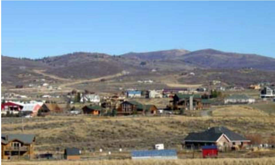
Inappropriate pattern for major development. Development should not spread across hillside.
